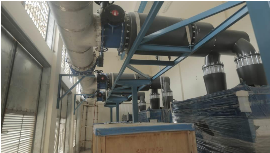
Structural and Mechanical Works for the Air Blowers in March 2019
