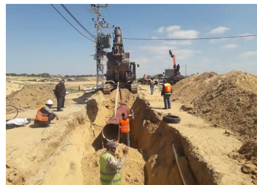
Ductile Iron Pipes Accessed to Gaza and Installed on Site for CMWU Package up to March 2019
