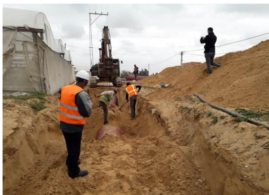
Ductile Iron Pipes Accessed to Gaza and Installed on Site for CMWU Package up to March 2019
