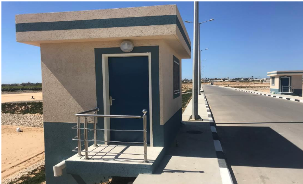
Accomplished Works of the Infiltration Basins before November 2018
