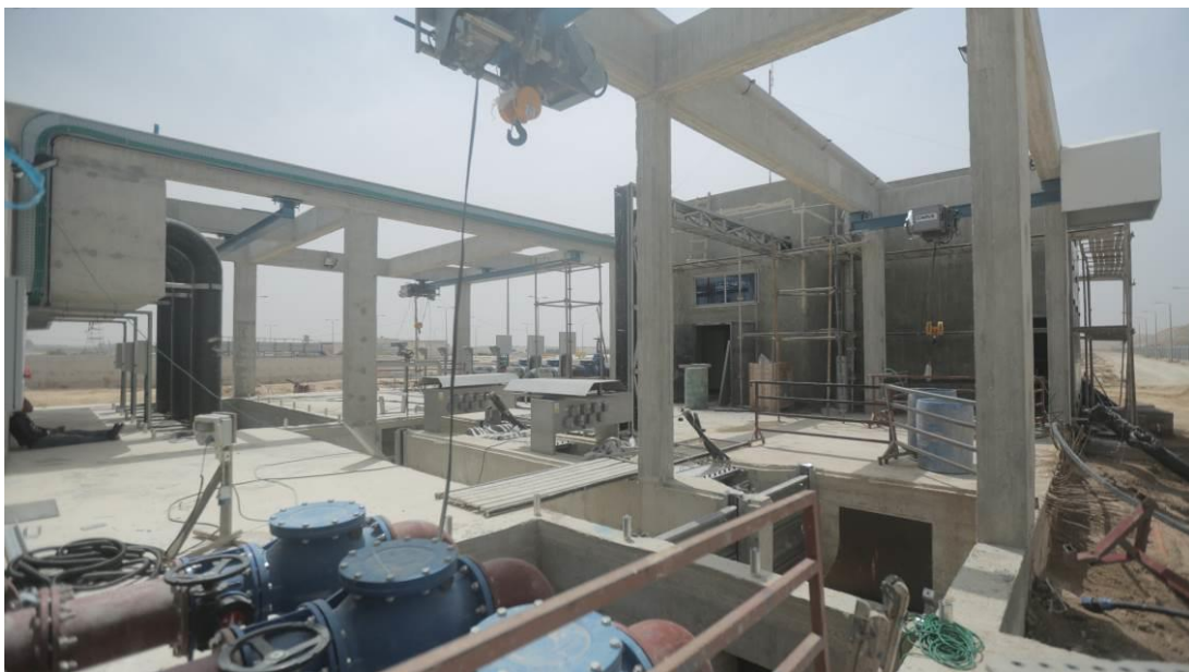
Structural and Mechanical Works for the Sand Filter in March 2019
