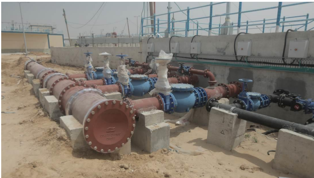
Structural and Mechanical Works for the Clarifiers in March 2019
