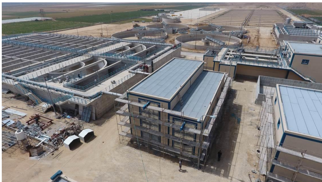
General View for Accomplished Works of KY WWTP in March 2019
