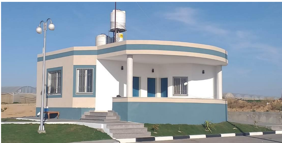
Admin Building for the Infiltration Basins up to March 2019
