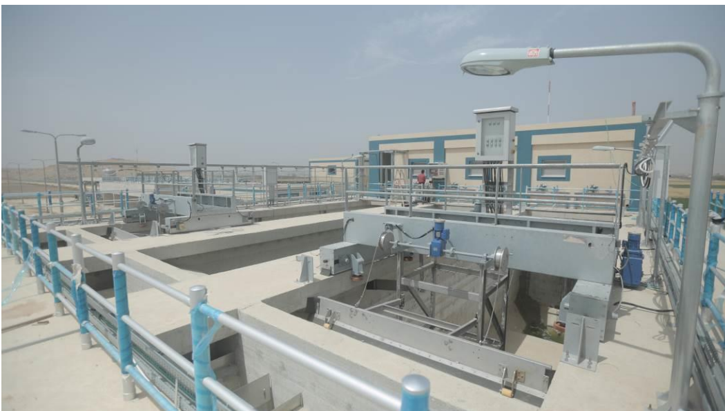
Structural and Mechanical Works for the Pre-Treatment Building in March 2019
